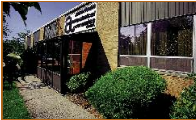
▲ ATC's New York Facility occupies approximately 90,000 sq. ft.
